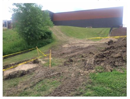
Site photo facing southwest illustrating the preparation of the pump pad (lower left) and treatment building foundations (middle right)
