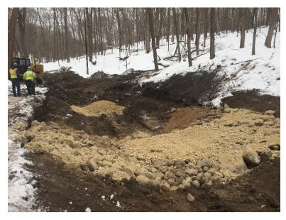
Beginning installation of a rock riffle toward the upstream end of the project
