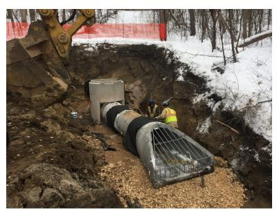
Installation of a storm sewer toward the downstream end of the project
