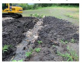
Additional Rock Riffle being install where headcut began forming this spring
