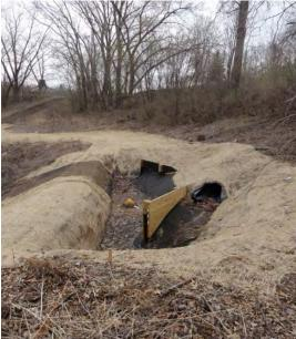
Spent-lime treatment system upstream of Wakefield Pond during construction before spent lime has been added.
