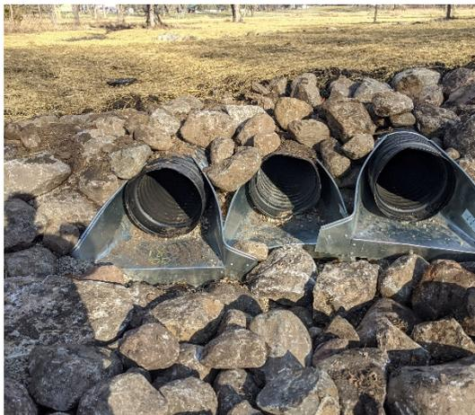
***Constructed flared end sections looking upstream from the ditch into the wetland.***
