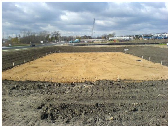
Construction of Beam Avenue iron-enhanced sand filtration system.
