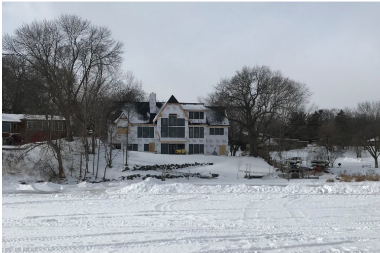
7300 Laredo Dr Chanhassen. Site condition on February 1, 2022.
