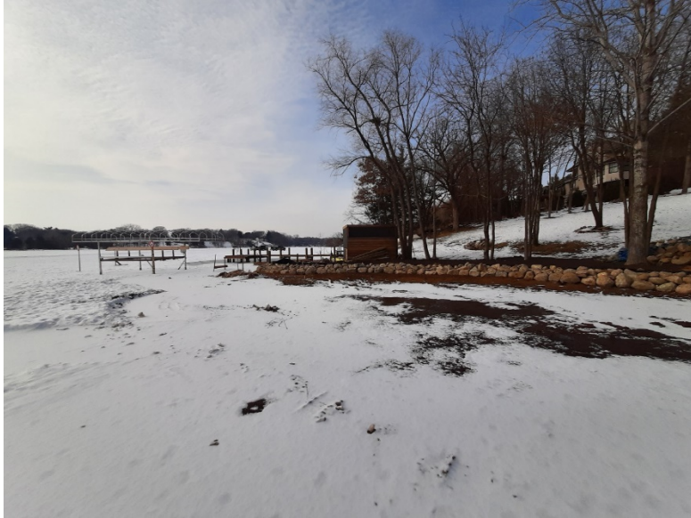
Riprap, fill, structure, and vegetation clearance at 15252 Boulder Pointe Rd Eden Prairie.
