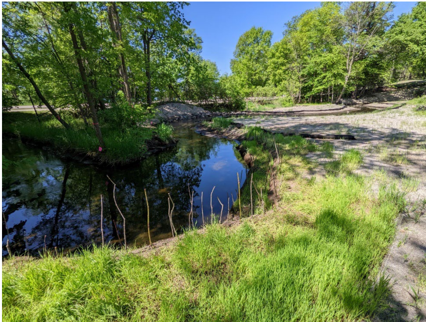
Photo of south site, looking upstream at VRSS and live stakes
