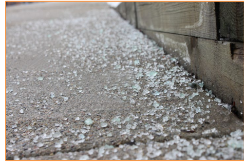
Figure 4-9 Heavy Salt Application
