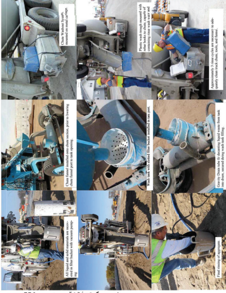
Approximately 1.5 times cycles are necessary to adequately clean the truck. The washout system is designed to capture washout water from concrete trucks. It consists of a concrete washout tank with a chute washout system and a 2" particle trap. Washout water is captured in the chute washout system and then flows into the concrete washout tank.
