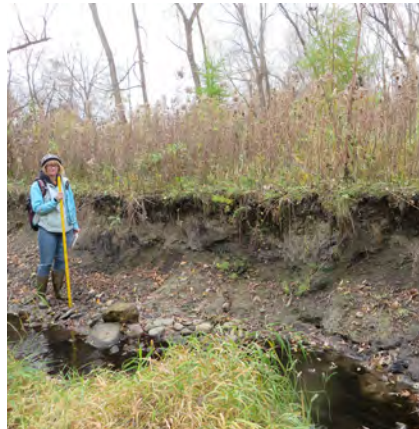
An eroded bank on Purgatory Creek that might benefit from stabilization.
