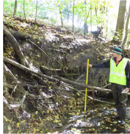
An eroded bank on Riley Creek that might benefit from stabilization.
