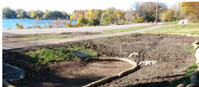
This large raingarden will catch and filter runoff before it enters Duck Lake. The photo was taken before the basin was planted.
