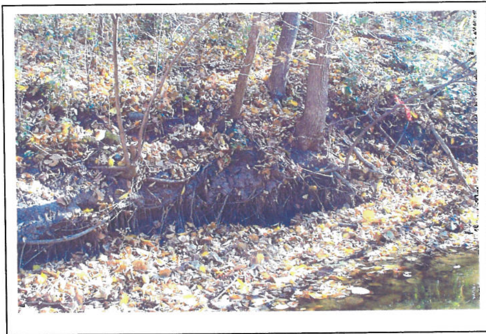
Figure PC16 – Reach P-3 Bank Erosion
