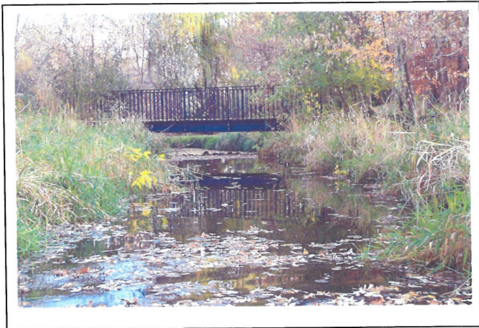
Figure PC22 - Reach P-5 Riprap Weir Below Pedestrian Bridge
