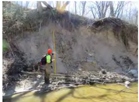
Measuring severe bank erosion along Bluff Creek
