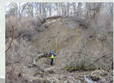
Left: An example of severe erosion. This eroded site was discovered during a field assessment as a part of the Creek Restoration Action Strategy.
