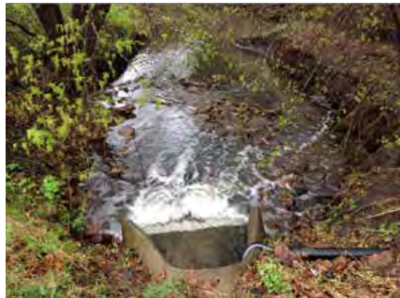
Stormwater discharging from Lake Susan Park Pond into Riley Creek
