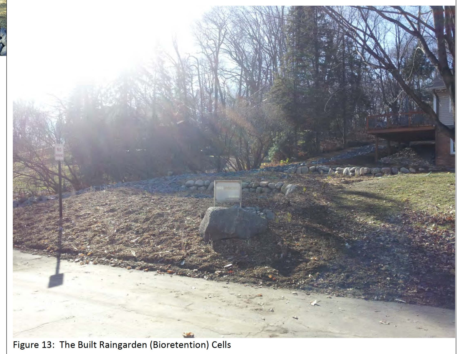
Figure 13: The Built Rain Garden (Bioretention) Cells
