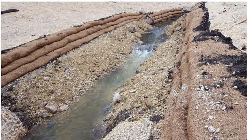
Constructed Riffle and VRS
