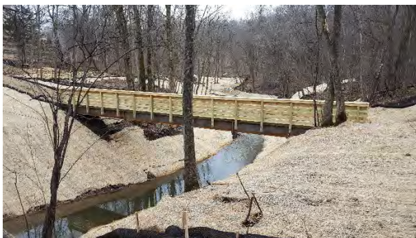
Installed pedestrian bridge
