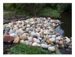
Photo of Riley Creek bank stabilization at Lake Susan Park Pond outlet
