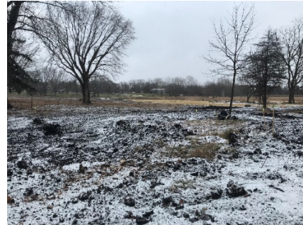
Partial straw mulch stabilization over excavated areas
