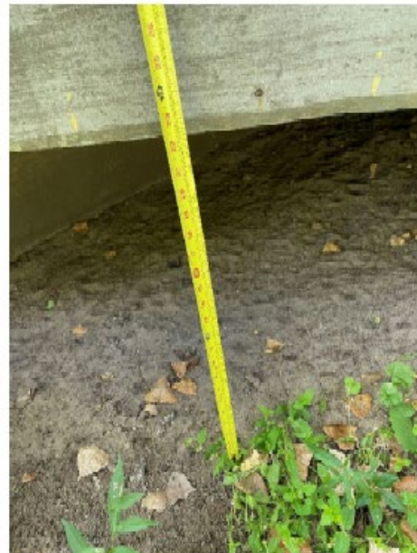
Sediment measurement in north culvert
