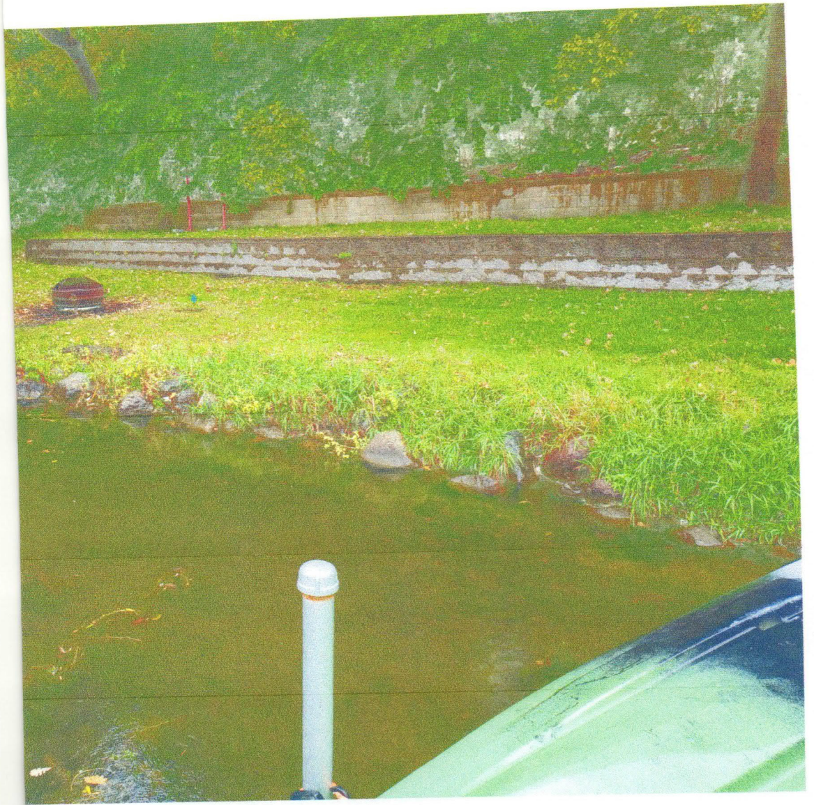
Existing riprap shoreline indicating erosion Prior to Construction.
