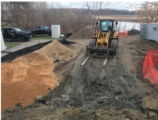
Project site looking south towards Rice Marsh Lake
