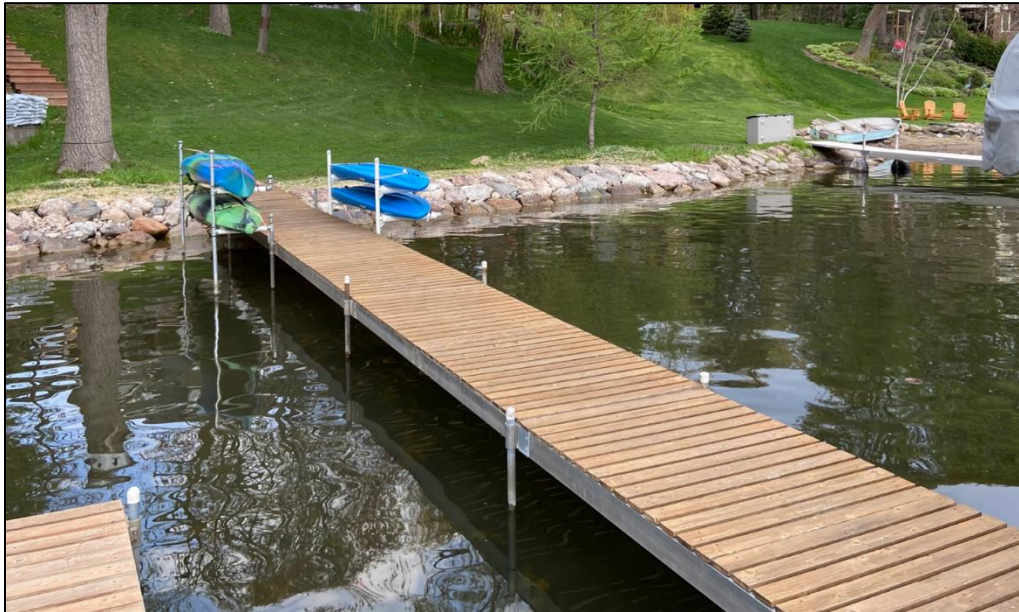
Figure 2. As-built Conditions with Neighboring Property in Background
