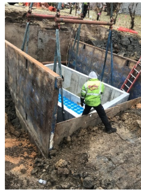
Installing one of the Kraken units
