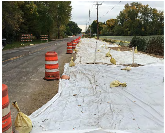
Covering exposed soils during road work reduces the risk of erosion into Duck Lake (fall 2021).
