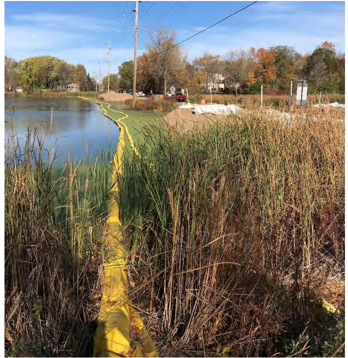
A double row of yellow silt curtains in the water protect the lake from the Duck Lake Road construction zone (fall 2021).
