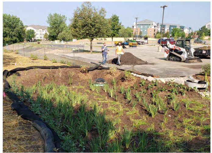
Photos taken during the installation of the St. Hubert Opportunity Project.
