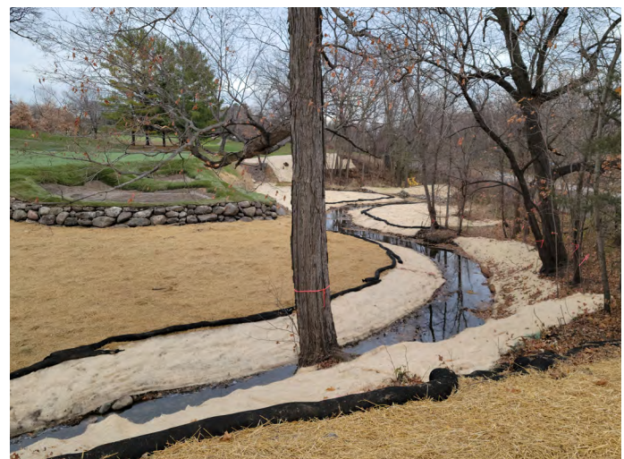
Re-meandering and bank stabilization of Riley Creek within Bearpath Golf and Country Club in November 2021.
