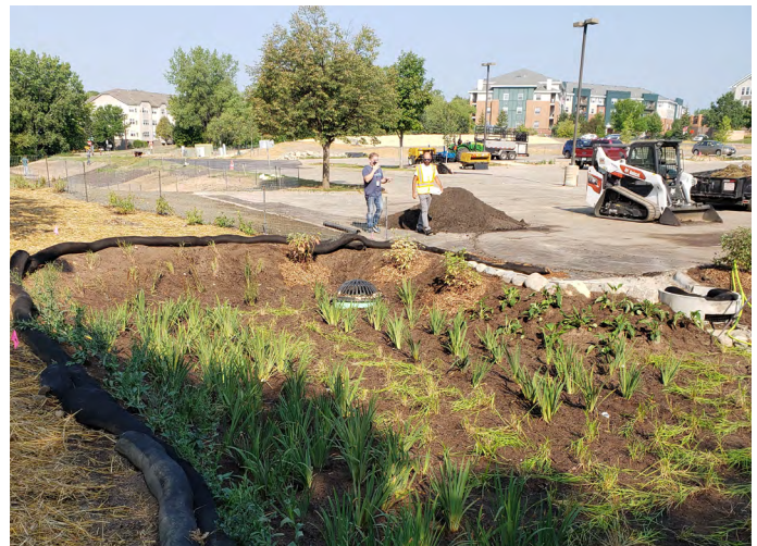
Photos taken during the installation of the St. Hubert Opportunity Project.
