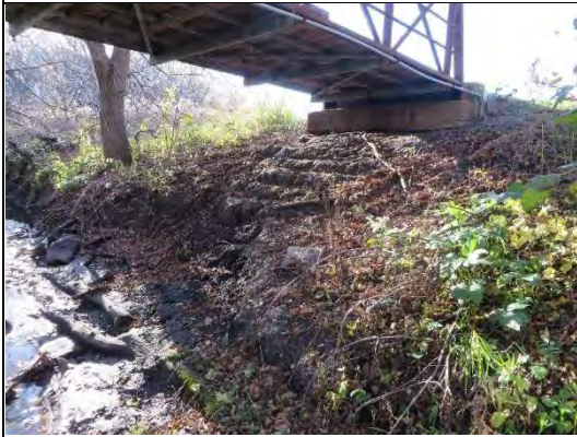
IMG-0225 Under IWOC bridge right bank
