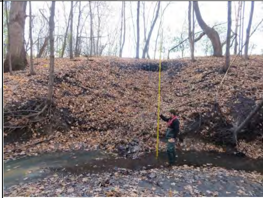
IMG-0234 Possible groundwater seepage area; causing erosion measuring 3.8m by 5m wide
