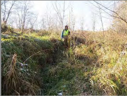
IMG-0257 Stormwater culvert channel entrance along right bank
