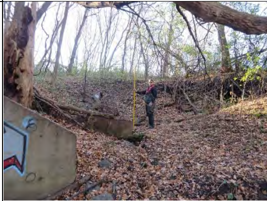
IMG-0238 Erosion from drainage on right bank; lots of dumped junk
