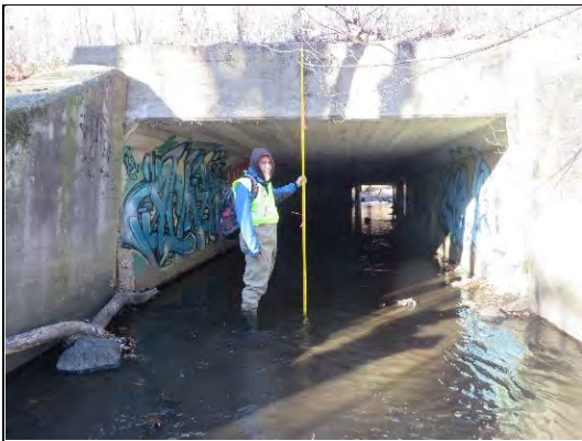
IMG-0240 Culvert under the railroad bridge (facing upstream)
