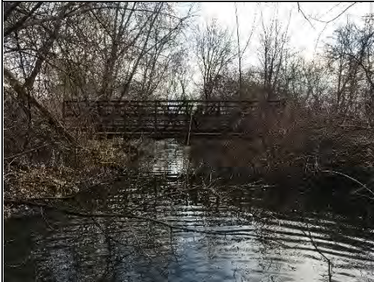
IMG-0339 Walking trail bridge over the stream
