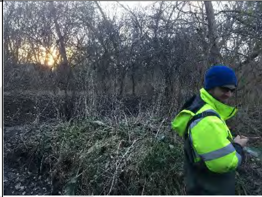
IMG-0327 Signs of major bank sloughing, partially healed over; right bank
