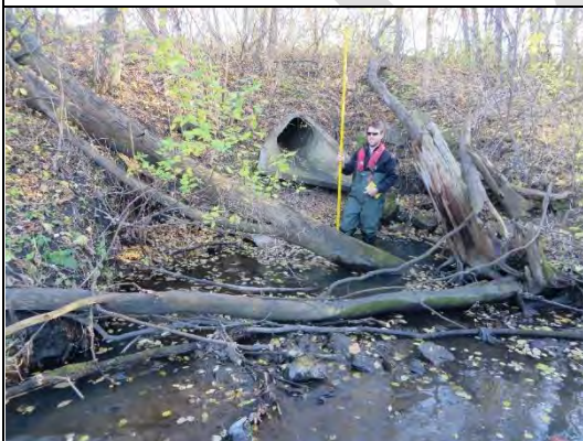
IMG-0229 Stormwater culvert on left bank, undercut 0.8m.
