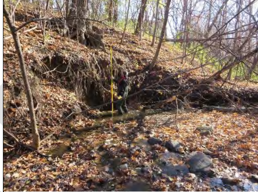
IMG-0186 Outside bend erosion on left bank, 2.2m by 8m
