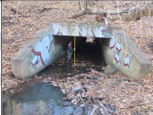
IMG-0236 Box culvert underneath the railroad bridge
