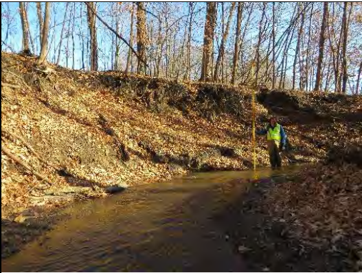
IMG-0255 Large erosion patch, 3.3m x 9m on right bank
