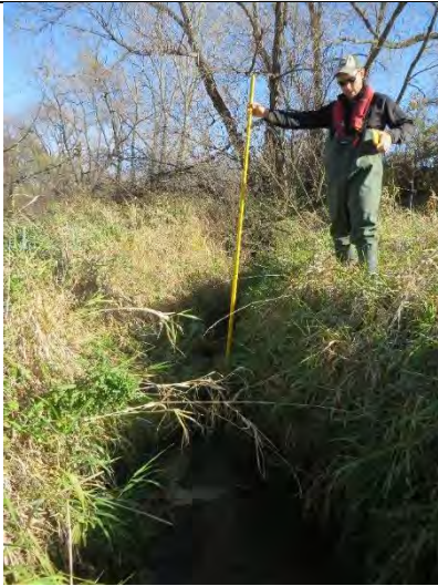
IMG-0208 Evidence of bank sloughing
