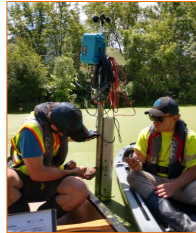
Figure 40 EnviroDIY Fixed Pond Continuous Monitoring Station
