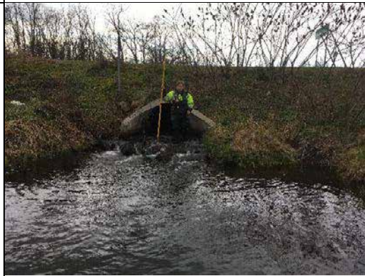
IMG-0349 Downstream view of culvert under Great Plains Blvd (facing upstream)
