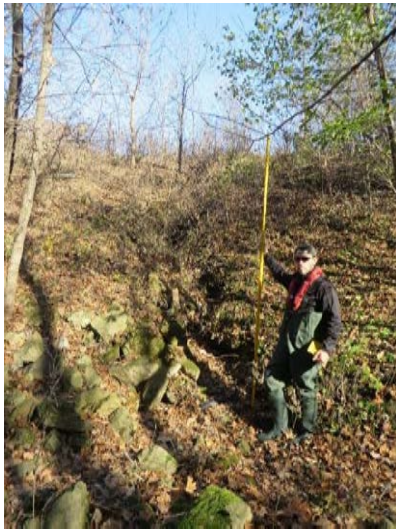
IMG-0185 Drainage from road causing small eroding ravine
