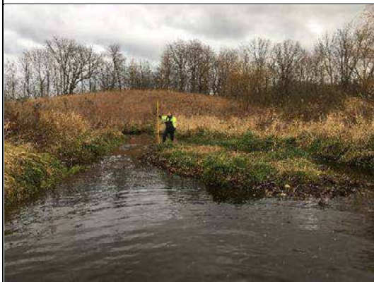
IMG-0351 Large grassy island below culvert
