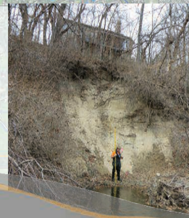
Left: An example of severe erosion. This eroded site was discovered during a field assessment as a part of the Creek Restoration Action Strategy.
