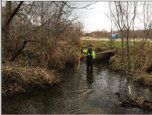
IMG-0347 Stormwater culvert left bank; Great Plains Blvd culvert
