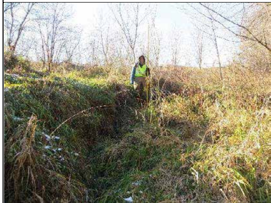
IMG-0257 Stormwater culvert entrance along right bank
