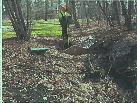
Photo 2: SW culvert top of side channel, mowed grass to edge.
