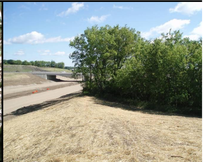
Figure 4.41 Highway 212 construction at head of ravine (Site 21)
