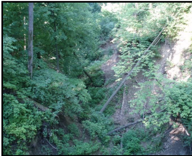
Figure 4.30 Looking down the ravine from golf cart bridge (Site 15)
