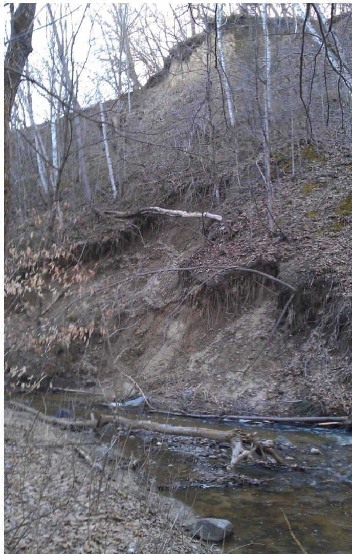
Figure 4.43 Example of main channel scarp along Bluff Creek
