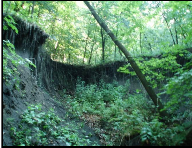
Figure 4.12 Large headcut in lower part of ravine (Site 6)
