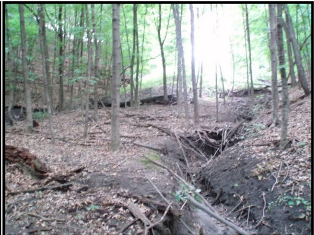
Figure 4.7 Headcutting in the Upper Part of the Ravine (Site 3)
