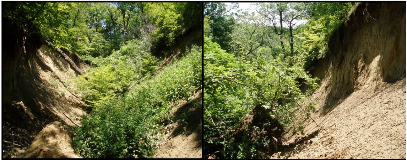
Figure 4.20 30-foot deep slope failure area (Site 10)
