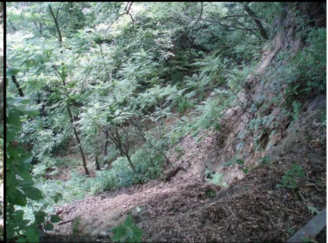
Figure 4.11 Yard waste dumping onto failed slope (Site 5)
