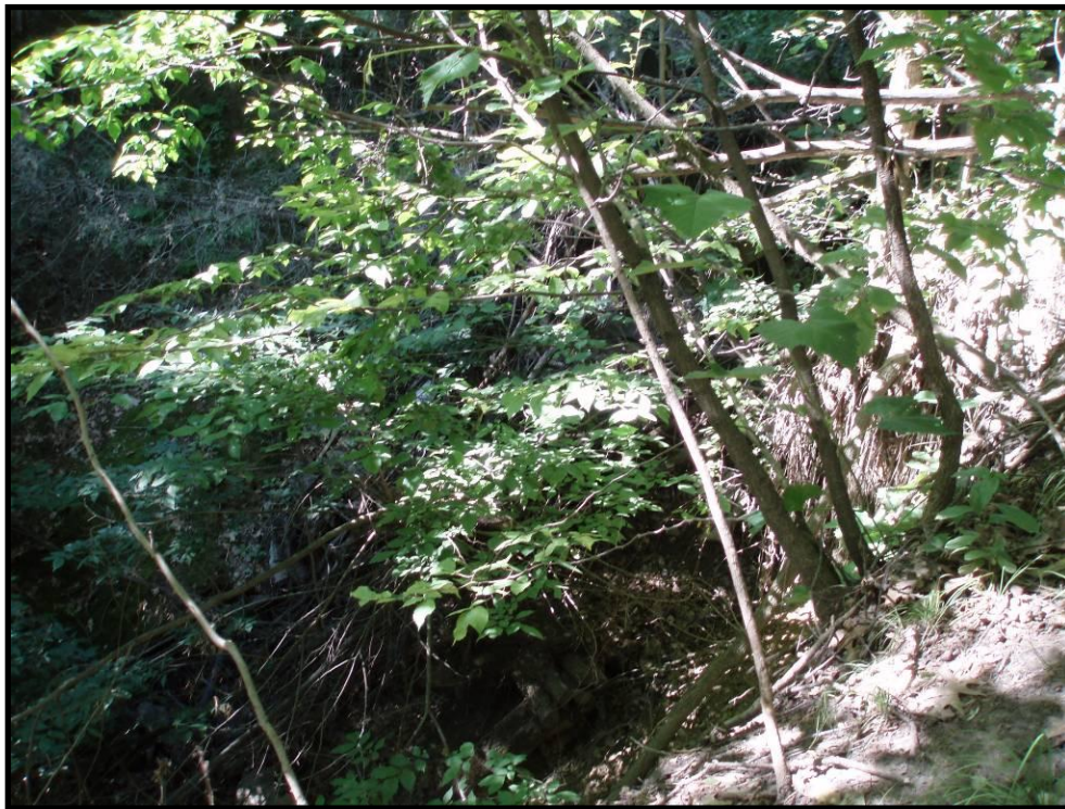
Figure 4.38 Slope failure near head of ravine (Site 19)
