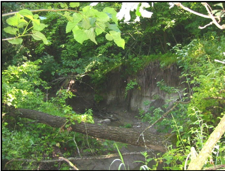
Figure 4.39 Bank erosion on outside of bend (Site 20)
