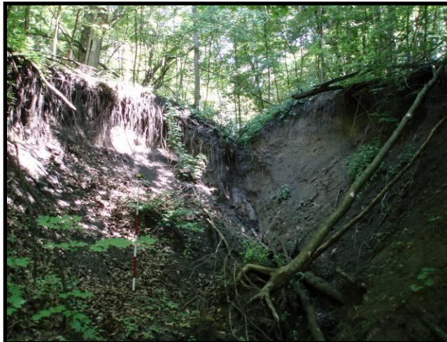
Figure 4.14 Large headcut in middle part of ravine (Site 7)
