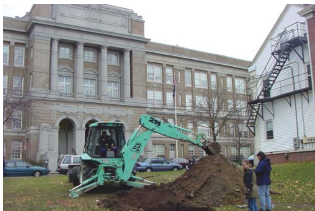
Figure 7.6: A backhoe used for digging a soil pit.
