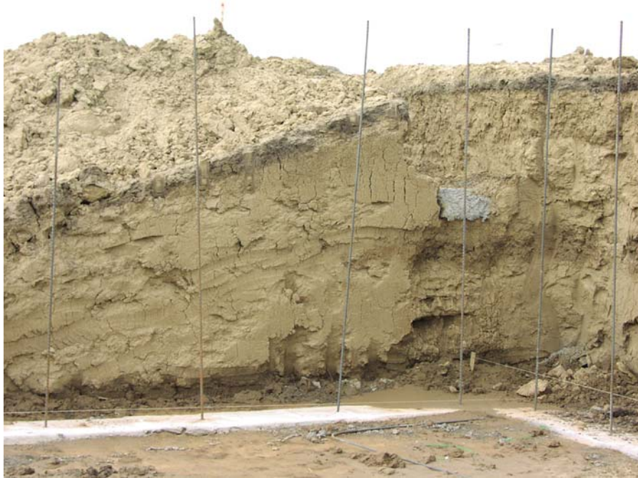
Figure 5.14: A filled area excavated for a home foundation.
