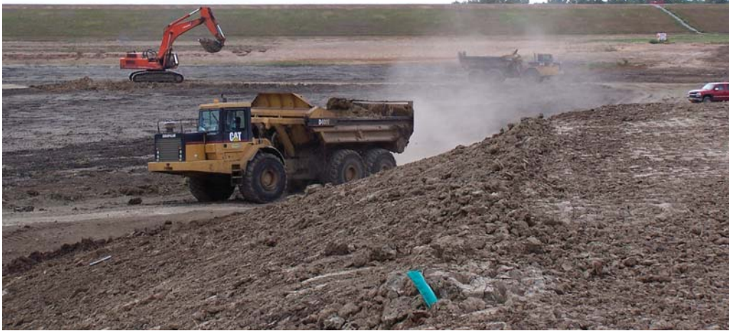
Figure 3.6: Removing sediment from a flood-control lake. A dam is in the background.
